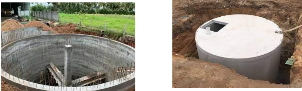
Fig.1 Cylindric water tanks construction
